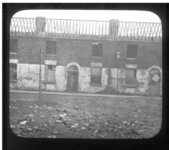
31 Glorney Cottages - typical low-value houses built in alleys off the main streets. Image from 1913, from Darkest Dublin slide collection [Photo: Royal Society of Antiquaries of Ireland]
