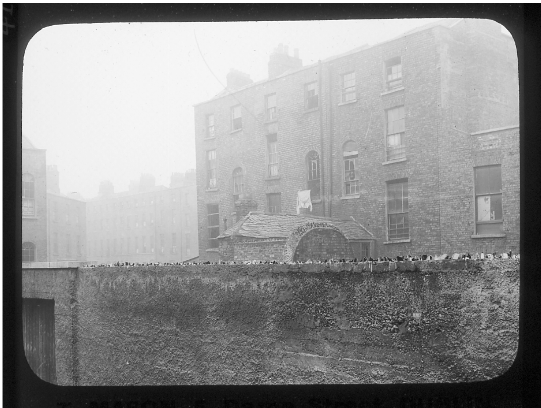
47 Gloucester Street Lower, showing the Diamond on the left, in 1913, from Darkest Dublin slide collection [Photo: Royal Society of Antiquaries of Ireland]. Note the poured concrete wall in the foreground, with broken glass bottles set into it.
